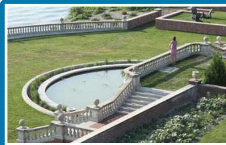
2012 saw structural repairs completed on the Lily Pool as part of the ongoing Formal Gardens Restoration Project.
