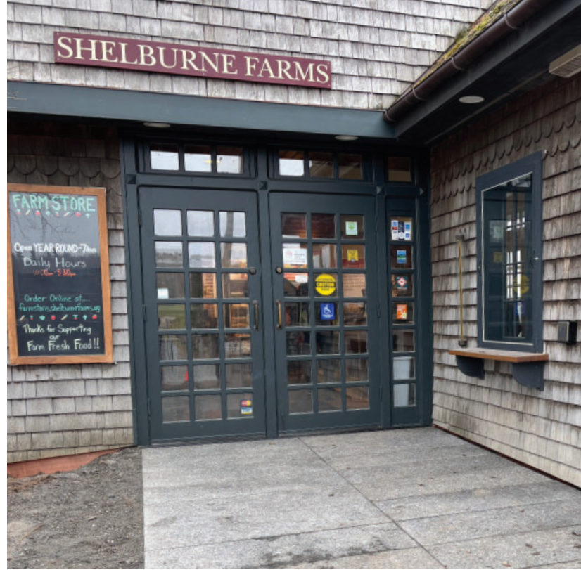
The Welcome Center has a new accessible entrance (bathrooms, too).
